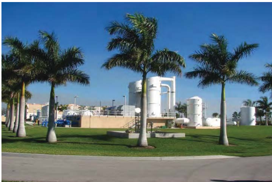
Water Treatment Plant No. 11, Belle Glade
