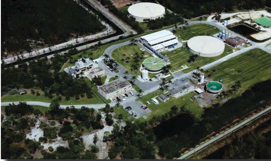
Water Treatment Plant No. 2, Lake Worth
