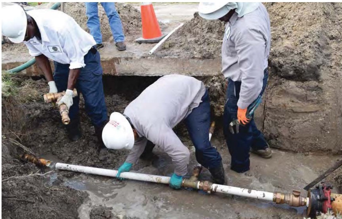
Northern Region Operations Center Line Crew, Royal Palm Beach
