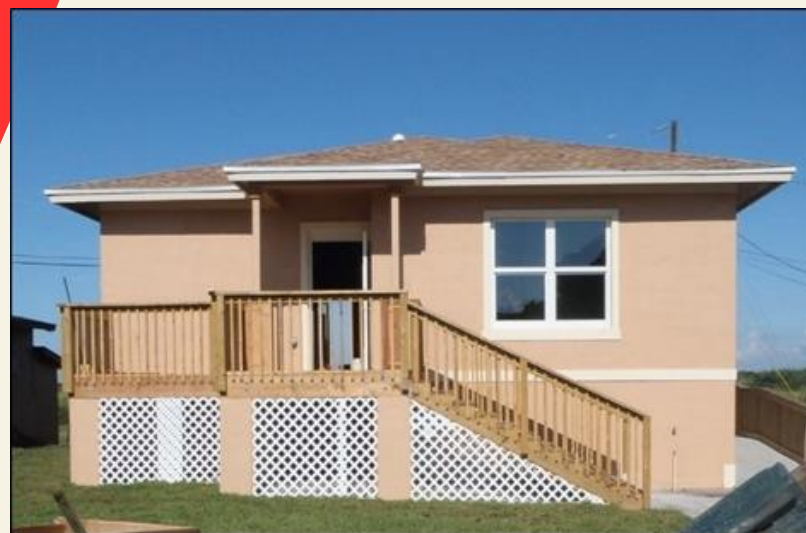
HED Replacement Housing South Bay
