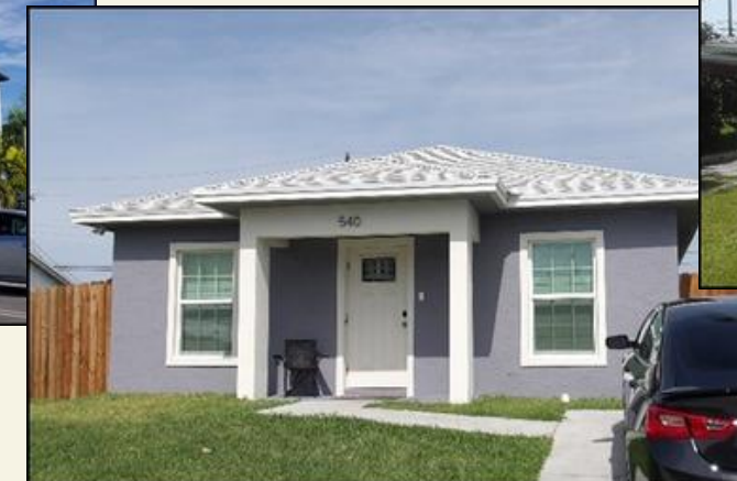
Habitat New Construction
