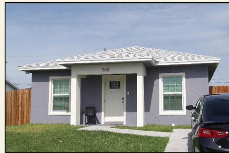
Habitat New Construction Belle Glade
