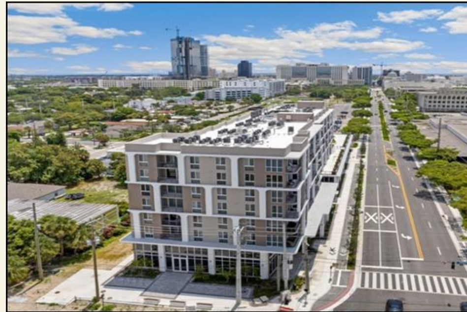
Flagler Station West Palm Beach 94 units
