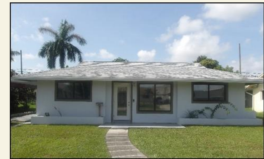
HED Housing Rehabilitation West Palm Beach
