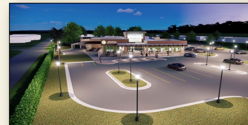
PBC/Gulfstream Goodwill Housing Resource Center II 74 Bed Emergency Shelter
