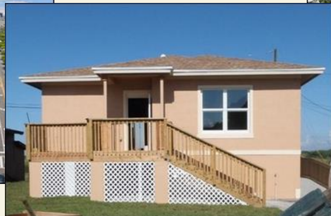
HED Replacement Housing
